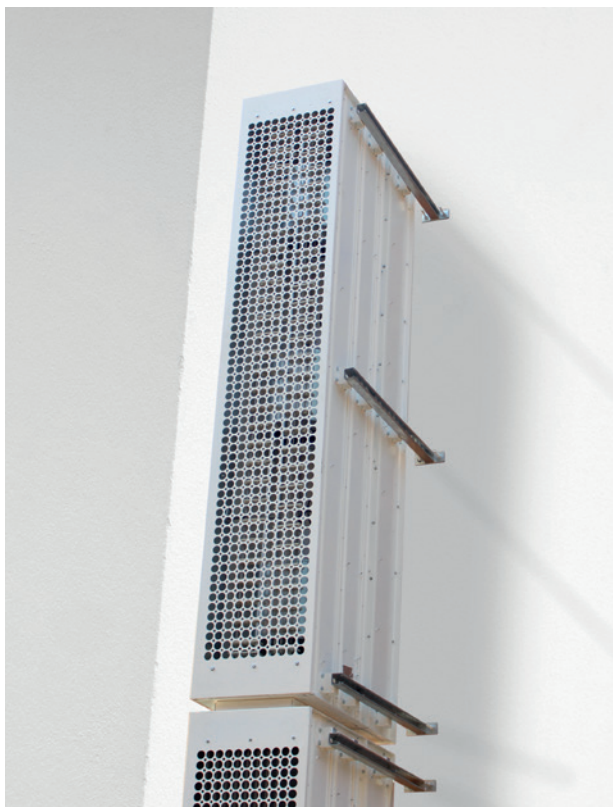
Vertically mounted stacked units via Unistruts and Vertical Mounting Plate
