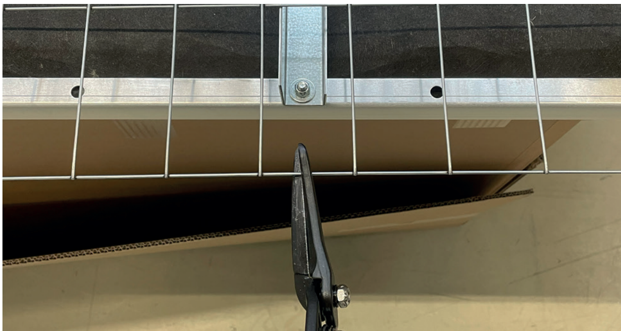
Figure 2. Snips breaking the mesh around the hanging brackets
