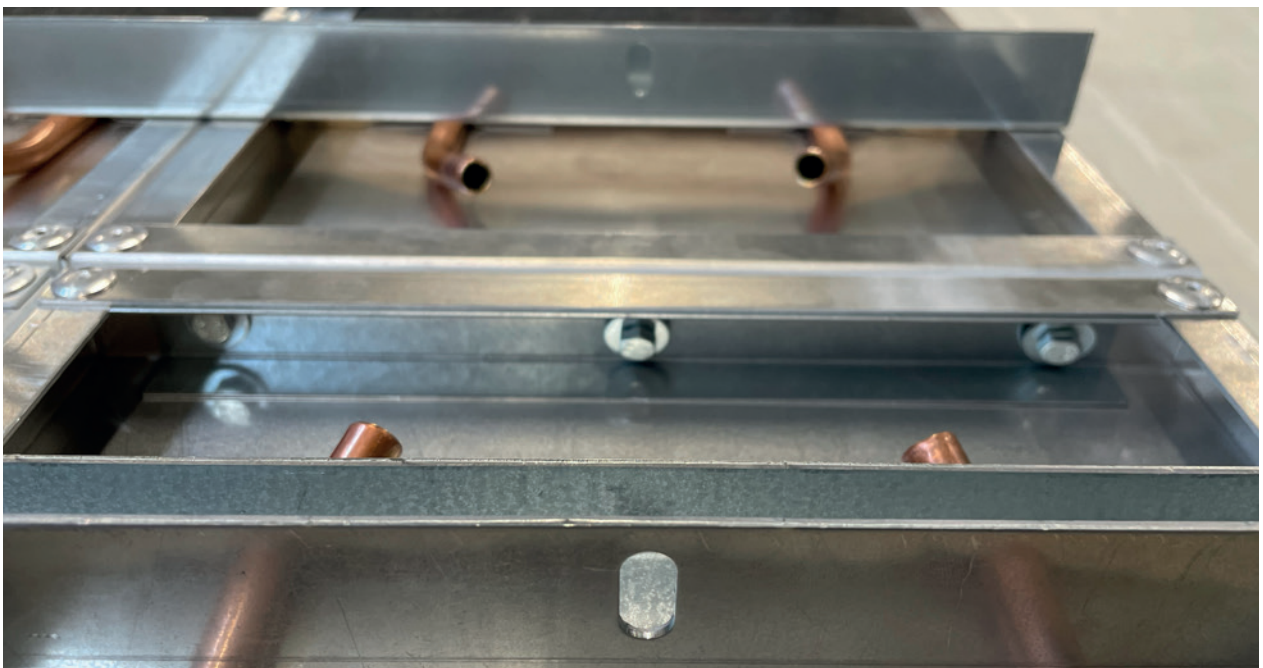
Figure 11. Adjacent panels screwed together via reinforcing channels
