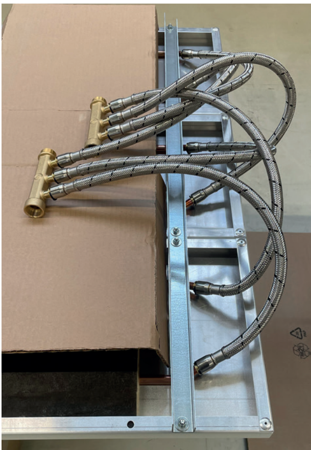
Figure 17. Flow and return manifolds and hoses
