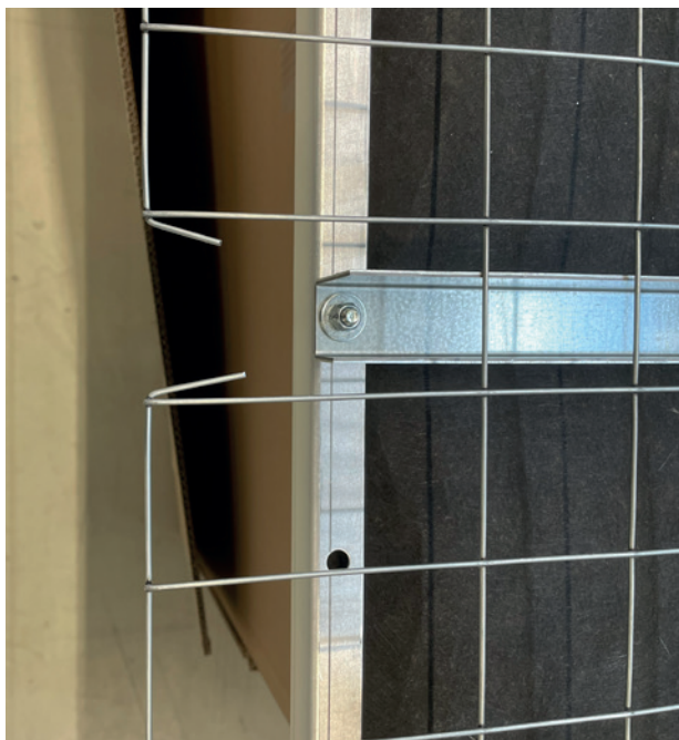
Figure 3. Mesh bent after snipping to avoid bracket when pushed inside flanges
