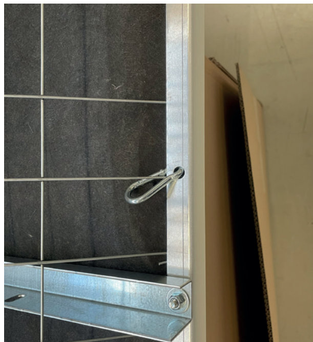
Figure 4. Carabiner clip holding mesh to side flange
