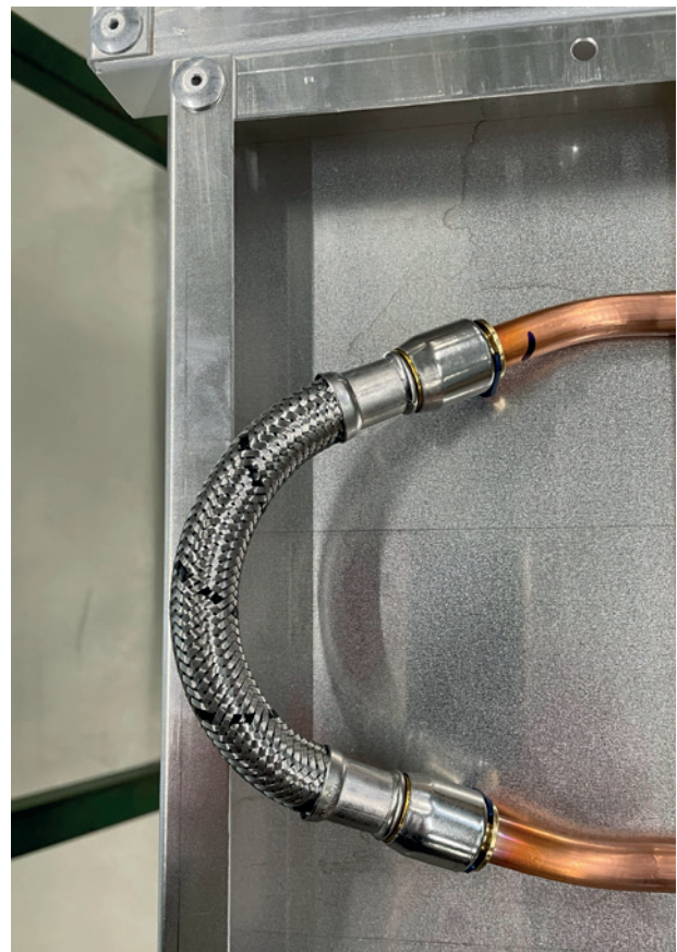
Figure 14. Return hose at end of panel run
