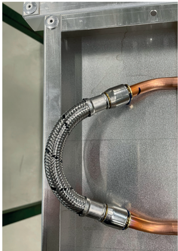
Figure 14. Return hose at end of panel run
