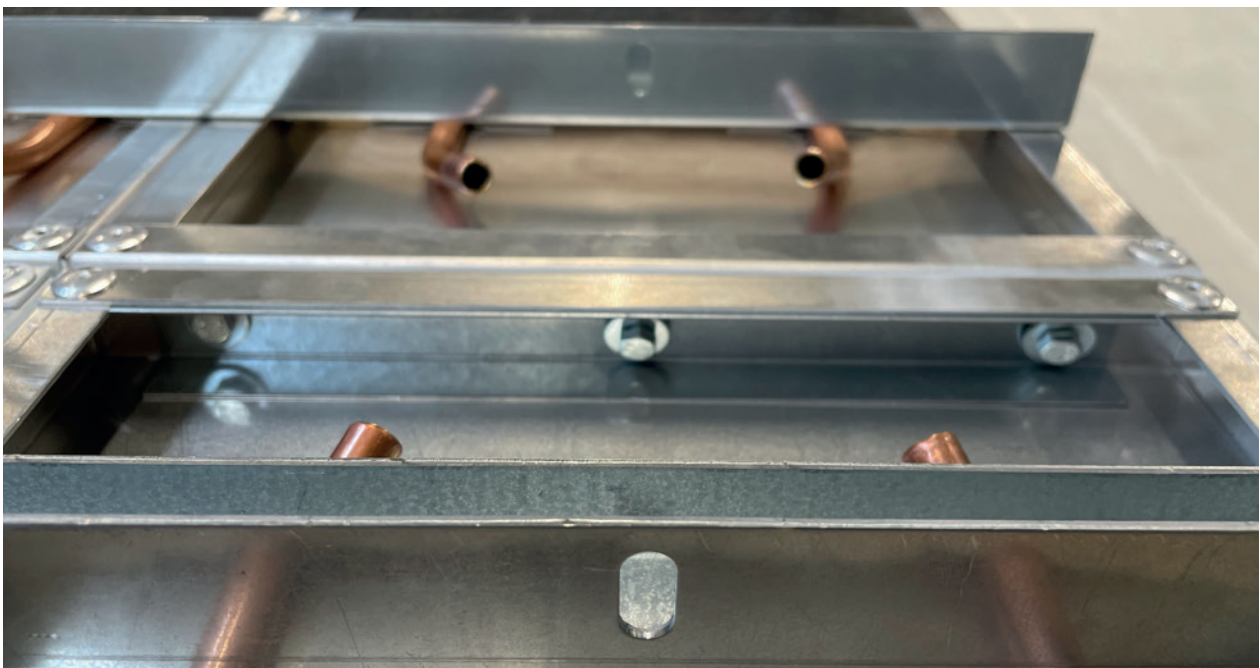
Figure 11. Adjacent panels screwed together via reinforcing channels
