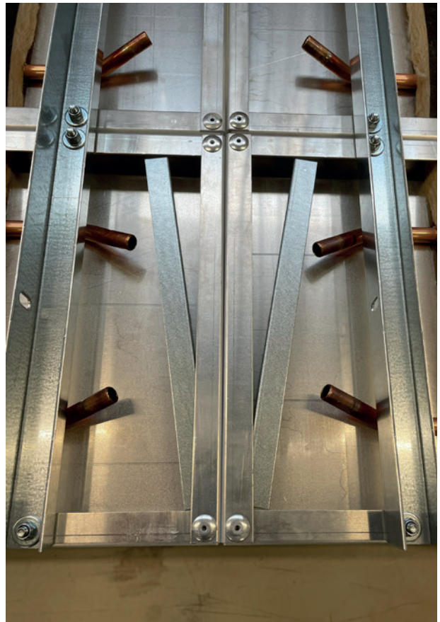
Figure 9. Reinforcing channels being slid into place
