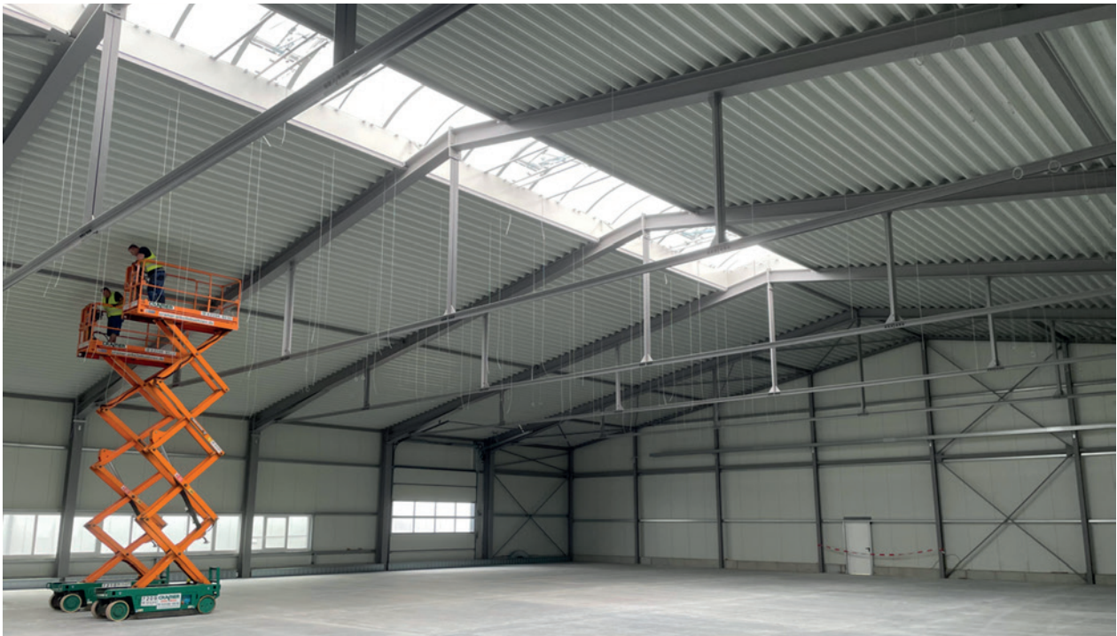
Figure 4. Suspension wires tied off from the ceiling
