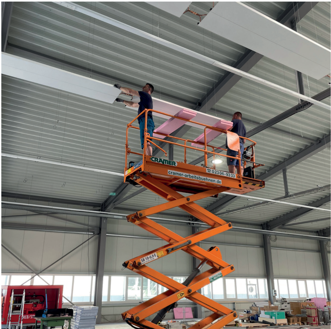
Figure 5. Scissor lift in use, note foam protection to prevent damage to the panels
